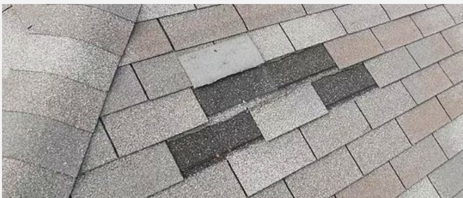
MISSING SHINGLES
